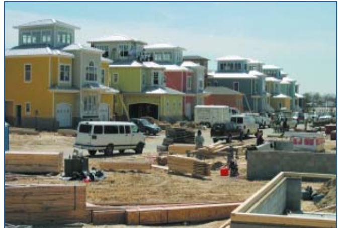
To justify the cost of a vacuum system, 150 to 200 connections are needed.
