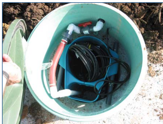
In a STEP system, an effluent pump is installed within a pump vault in the outlet end of a septic tank.
